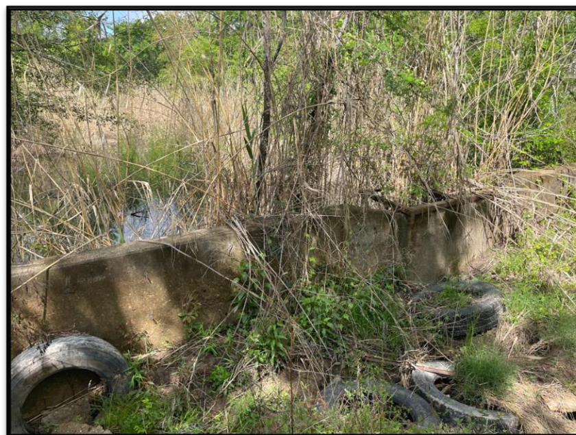
Site Photograph 2. Photograph taken near existing dam along drainage. (Photograph Date: 3/22/2024)
