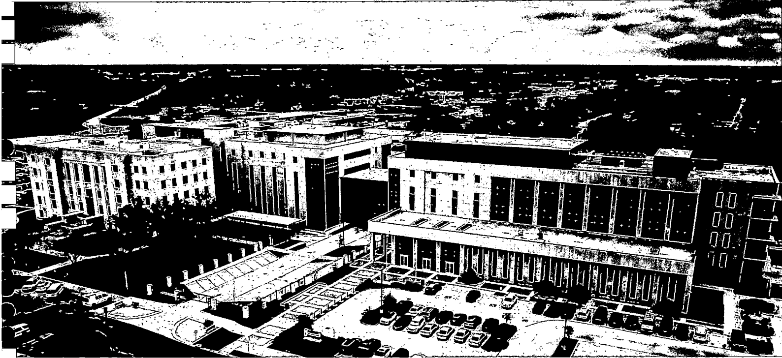
Brazoria County Courthouse Campus Expansion
