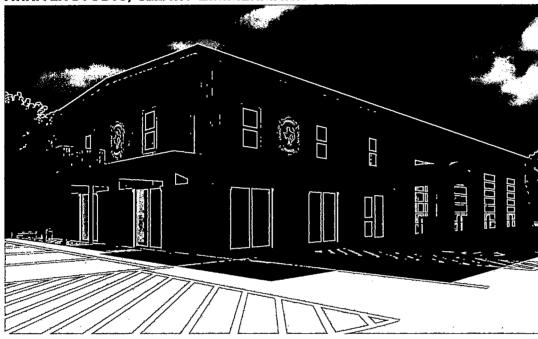
Addition and renovation of an existing 1970's pre-engineered metal building fire station. The addition includes two new apparatus bays on the West end of the building. The renovation includes the replacement of the building façade, all windows, as well as site improvements such as new concrete parking lot, preengineered metal building canopy, and brick street sign.
