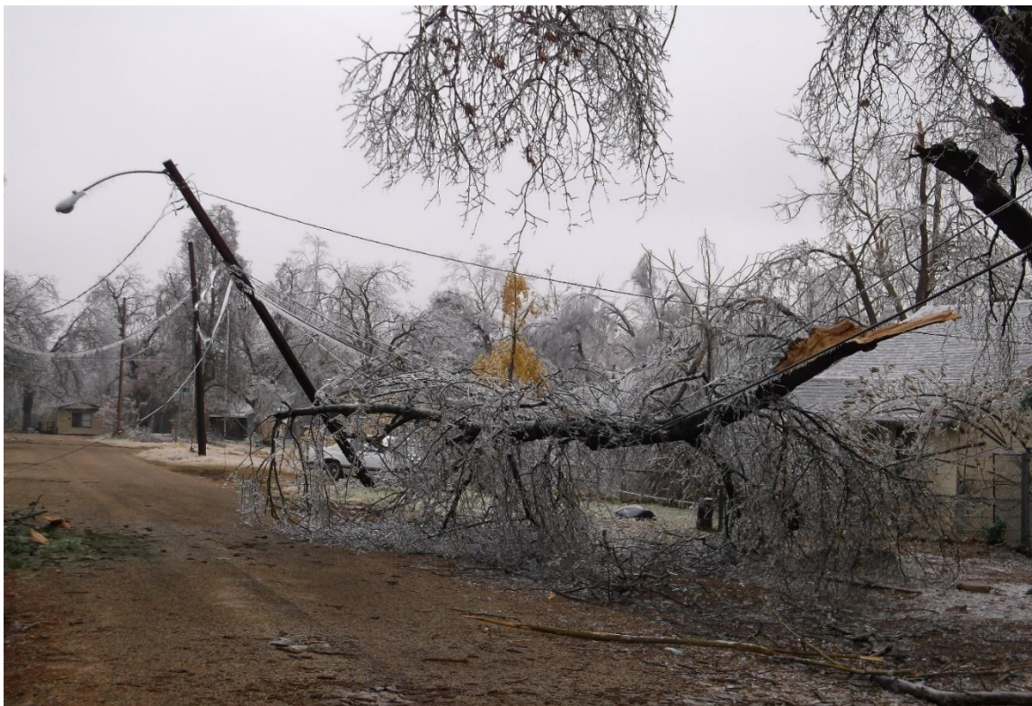
Figure 2-58: Downed power line during the 2013 ice storm in Paris, Texas. 330
